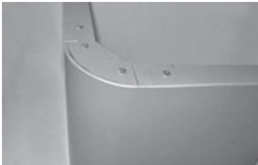
Corner Panel with Gusset and Filler Plate
