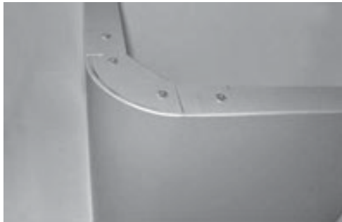
Corner Panel with Gusset & Filler Plate
