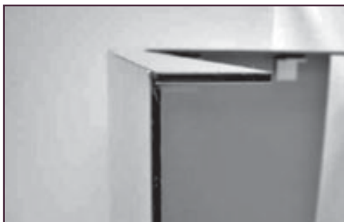
Cope at Edge of Panel
