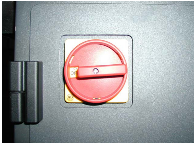
Main disconnect switch in the Off position
