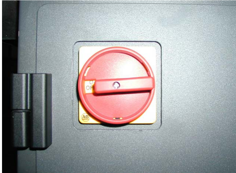
Main disconnect switch in the Off position
