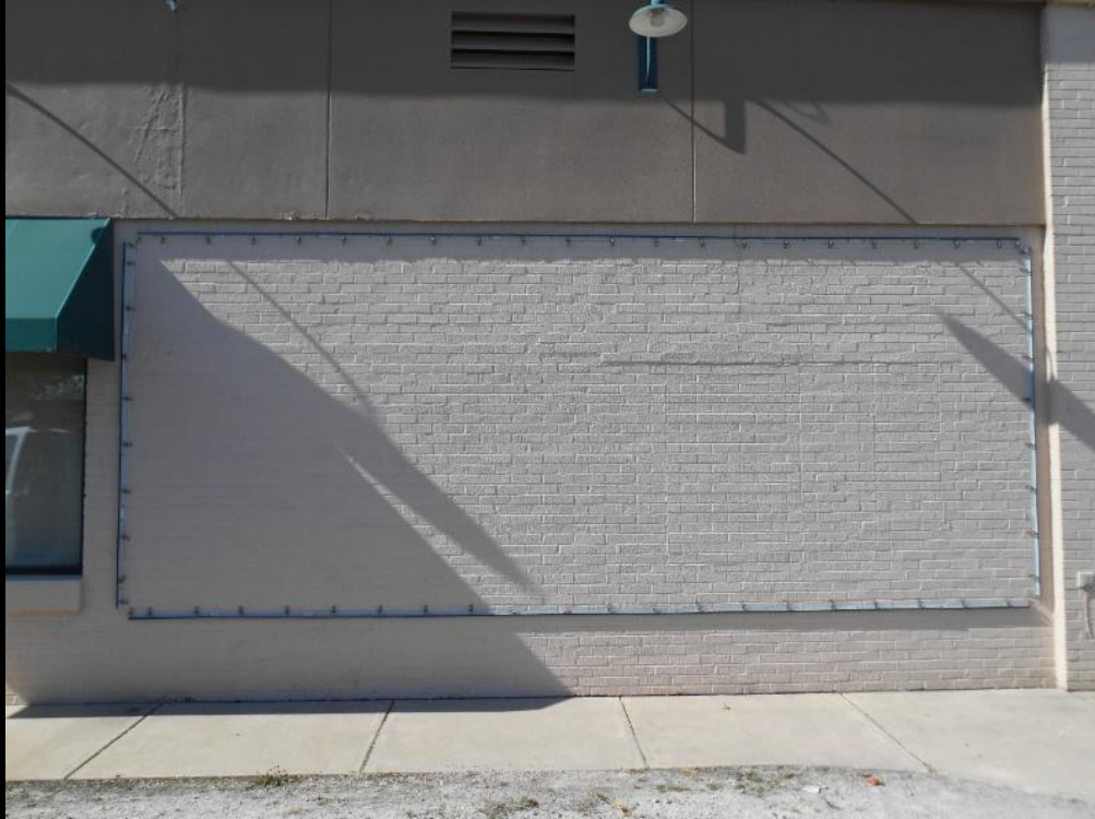
BannerFrame base channel installed 1.5" off the banner perimeter
